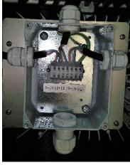
Connect the cables to the terminal board belonging to the driver plate
